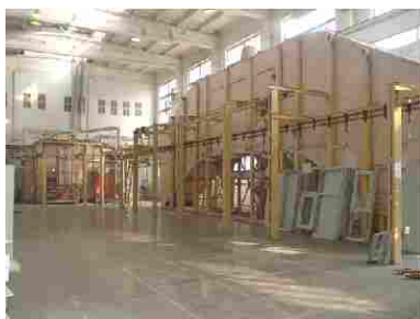
The powder painting line for metalworks
