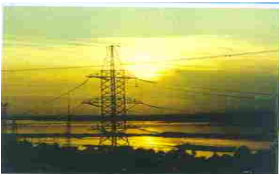
Electric power lines 750 kV
